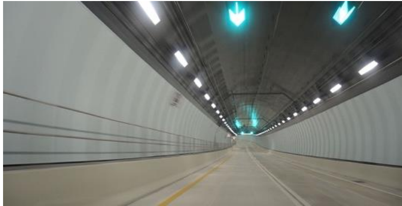
Photo 1 Port Miami Tunnel
