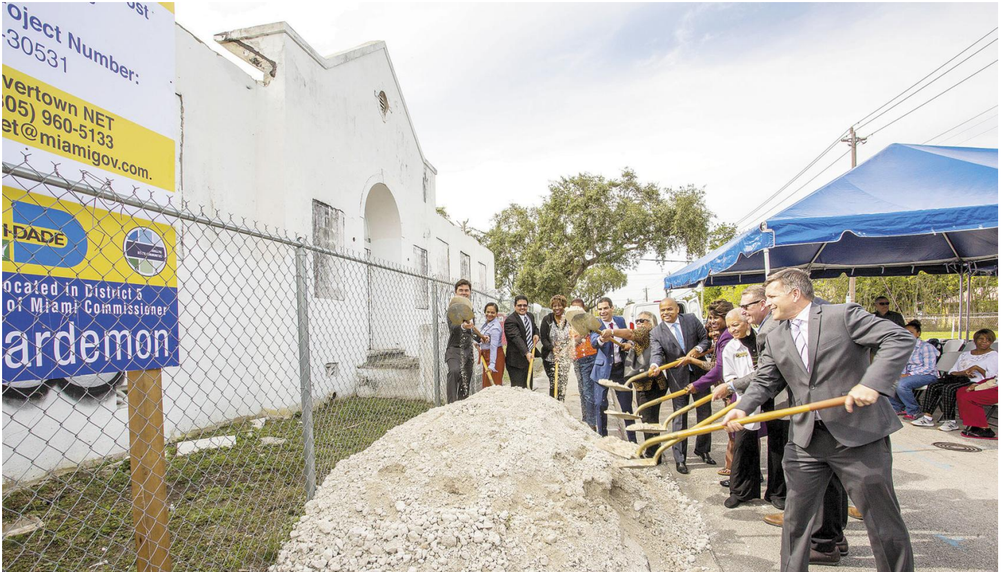
City leaders, relatives of D.A. Dorsey and Overtown residents lift dirt in ceremony for launch of the library renovation project.
