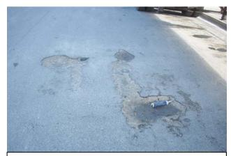
Damage to roadway along NW Miami Court as a result of heavy truck traffic.
