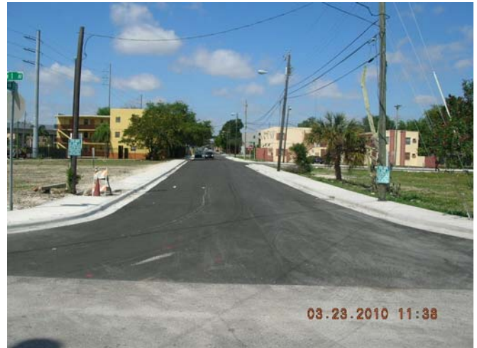
Road improvements along NW 11 th Terrace between NW 1 st Avenue and NW 1 st Place included new asphalt, and sidewalk installation.
