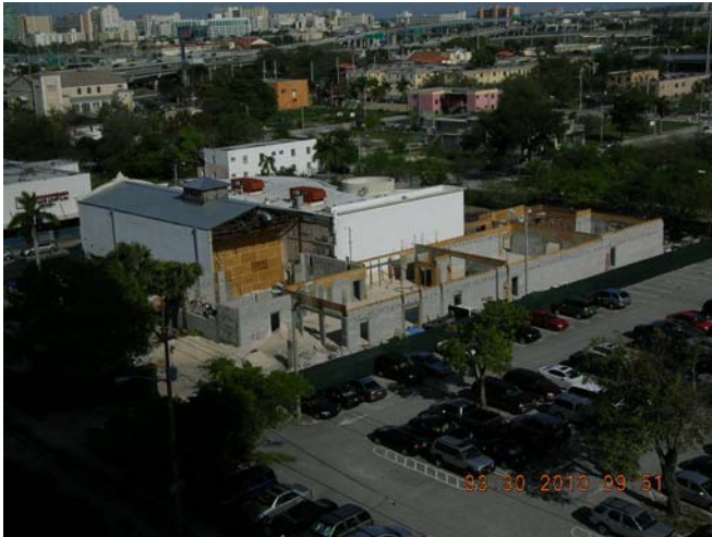
Ongoing construction at the historic Lyric Theater at 819 NW 2 nd
