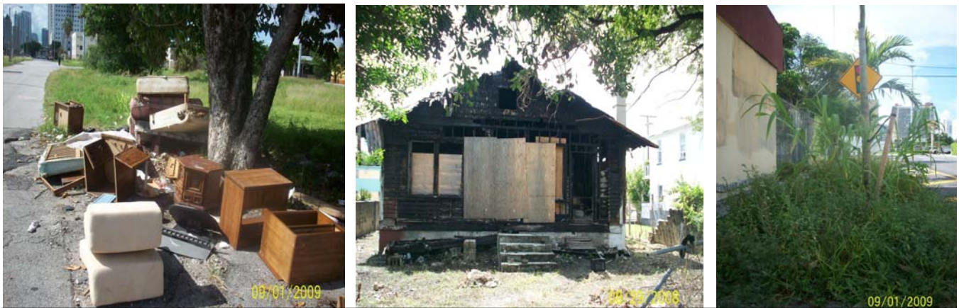
The Community Redevelopment Agency works closely with the City of Miami’s Code Enforcement Department and Miami-Dade County’s 3-1-1 service to ensure property owners comply with the local zoning and building regulations. The images above and below reflect the type of code violations prevalent in the Redevelopment Areas.
