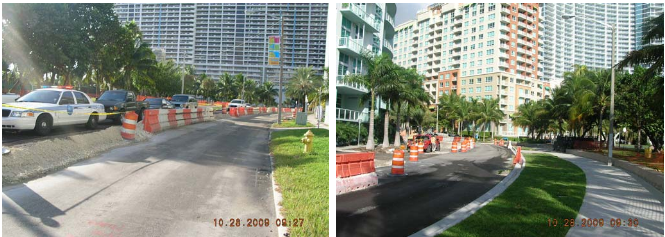
Road improvements along N.E. 17 th Terrace in Omni.
