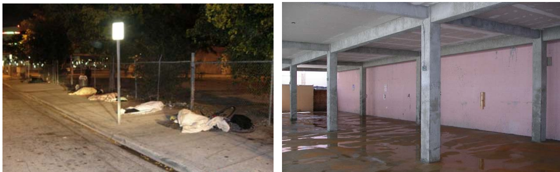
The CRA funded the construction of a covered shelter within the Camillus House at 726 N.E. 1 st Avenue.
