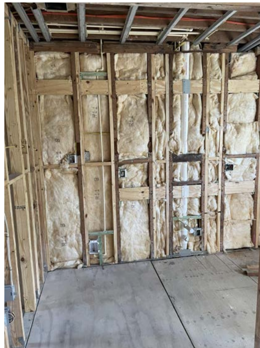
After - down to the studs, new plumbing, floor, electrical, insulation...
