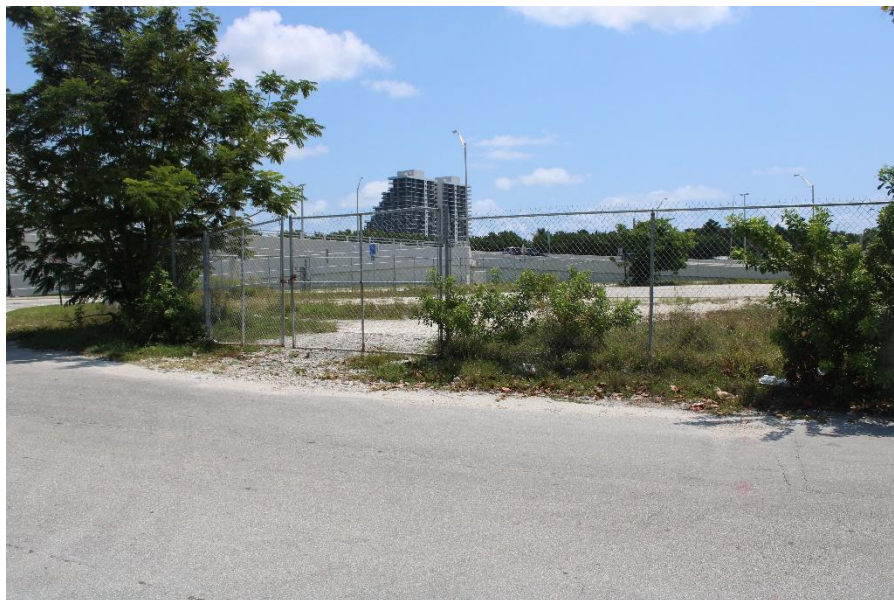
Exhibit: A large site on Watson Island demonstrates clear site deterioration to the visitors travelling along the McArthur Causeway.
